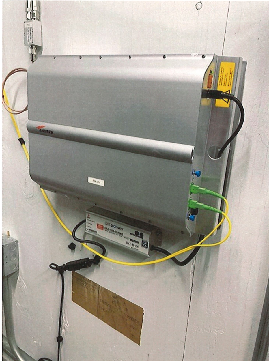
Distributive Antenna System (DAS) Repeater
