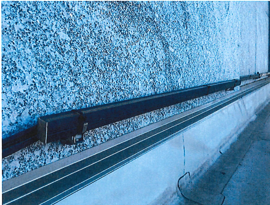
Existing LED lighting fixtures at Court's parapet that have failed and require replacement.
